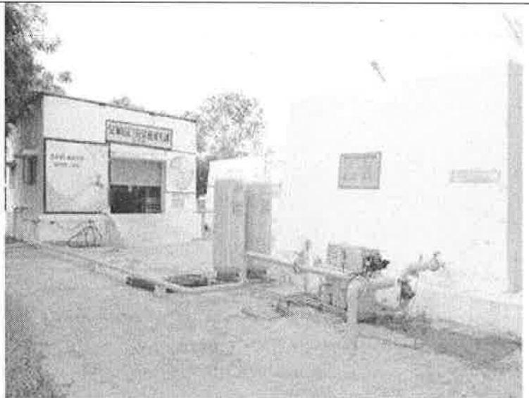
Sewage Treatment Plant
