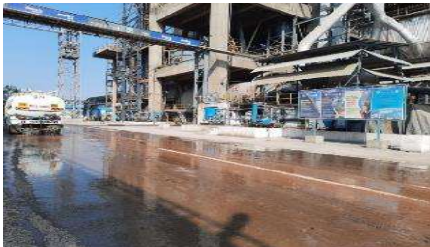
Water Sprinkling on Roads
