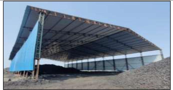
Coal Covered Shed
