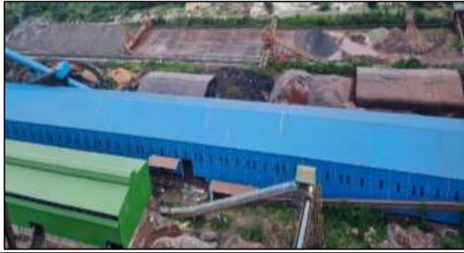
Raw Material Covered Shed
