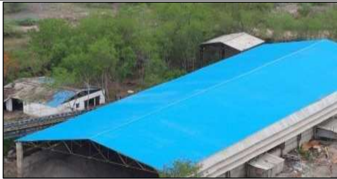
Gypsum Covered Shed
