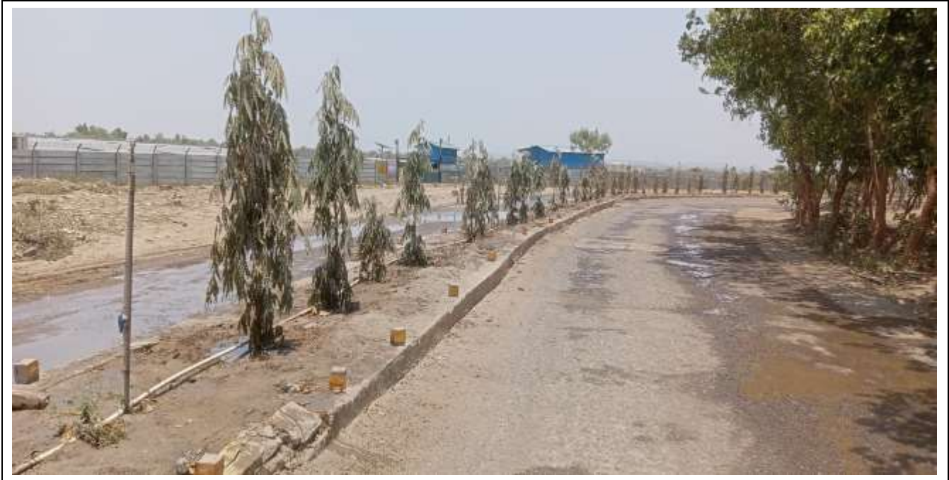
Water Sprinkling System along the Road
